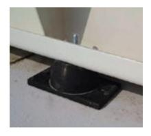
The antivibration elastic mount **Vibro EM.3** can be used to absorp vibration in air handling units, air conditioning units, pumps, air compressors, ventilatiors, transformers, motor generators, cutting machines, printing machines, lifts, etc. especially when machine fastering is necessary.
