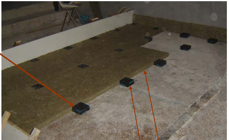
Double layer of VIBRO-EP 12.5x12.5x5cm Interstage layer of rockwool
