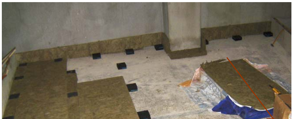
Rockwool or polyethylene expansion foil to avoid sound-bridge with the wall.
